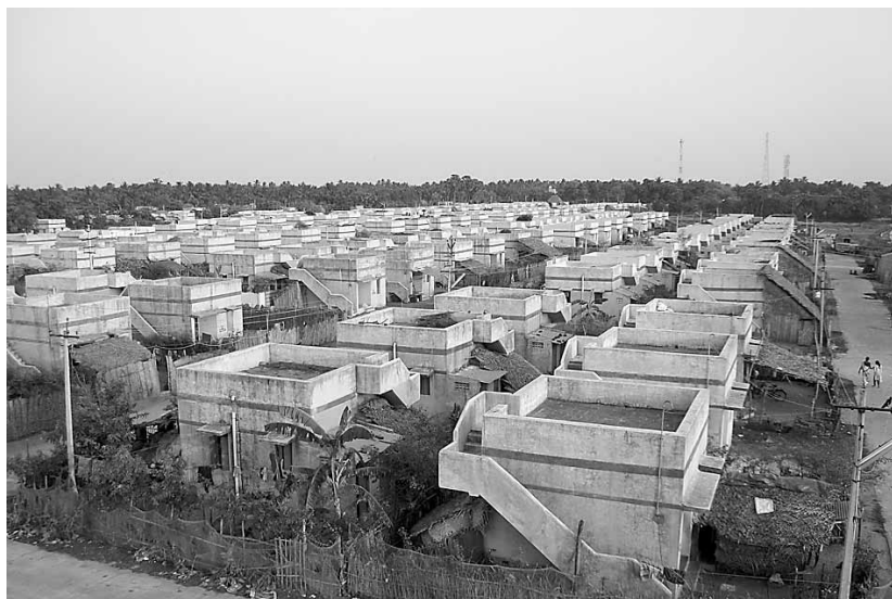
A complex of 525 disaster-resistant houses built with DWS/LWSI support, targeting fishermen and other marginalized communities including Dalits and members of scheduled tribes.
