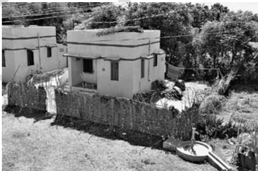
The LWSI-constructed houses offer better protection against cyclones, earthquakes and floods. © LWF/D.-M. Grötzsch
