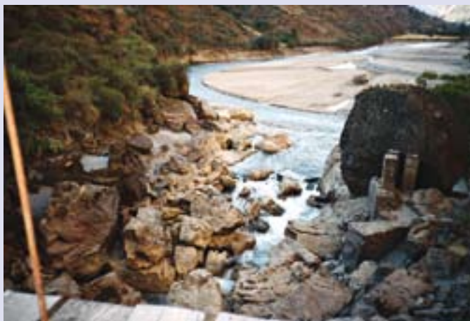
The canal's construction was a joint effort between the local authorities, community members and Diaconía – Peru. © LWF/DWS Peru/L. Hokkanen
