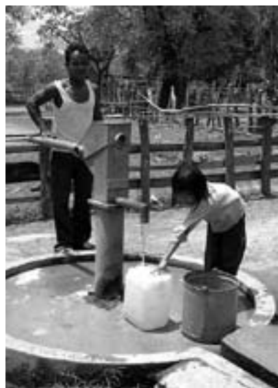
Built with LWF assistance, this well generates up to 4,300 liters per hour. The Suoy people fear the “eco-tourism” project could exhaust the underground water in the future. © LWF/D.-M. Grötzsch
