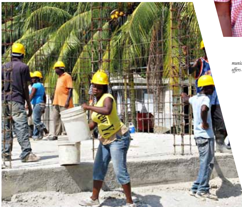
One year after the earthquake, reconstruction near Port-au-Prince. © LWF/Anli Serfontein
