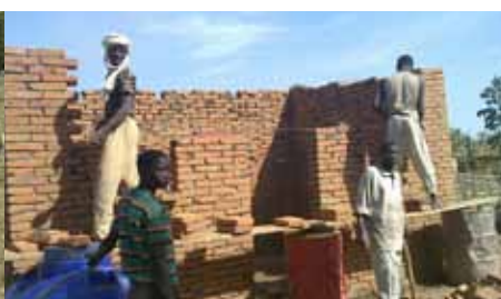
Amelioration of shelters for the vulnerable people in the IDP's villages
